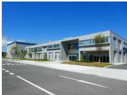
[Development Base Area] Research Building
